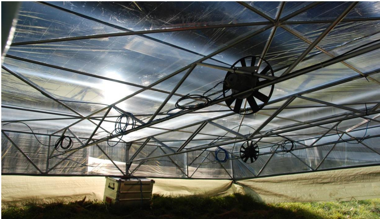
Figure 6: Inside of the large chamber. Ventilators and sampling tubes can be seen.
