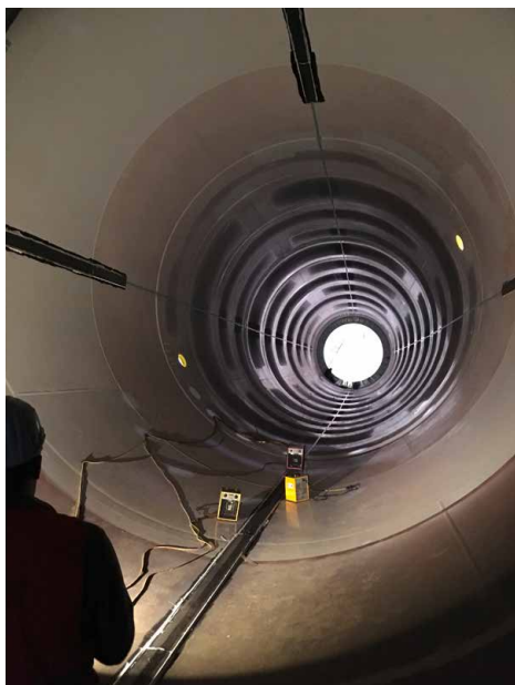
This Side: Instrumentation inside a Monopile (Photo IGB) Rock Salt after load test (Photo IGB)
