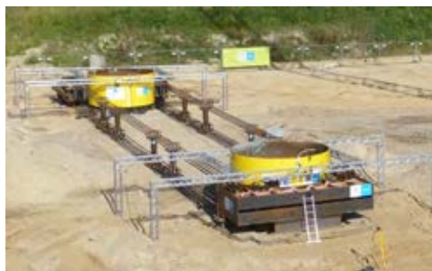
Test site in Cuxhaven © VIBRO-project
